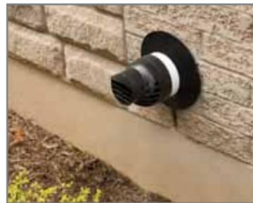
*The single concentric vent acts as both an air intake and exhaust, greatly simplifying installation.*
